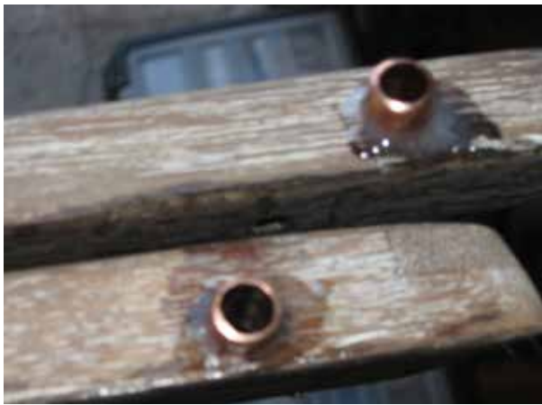
windows received new weep hole drains expoxied in place
